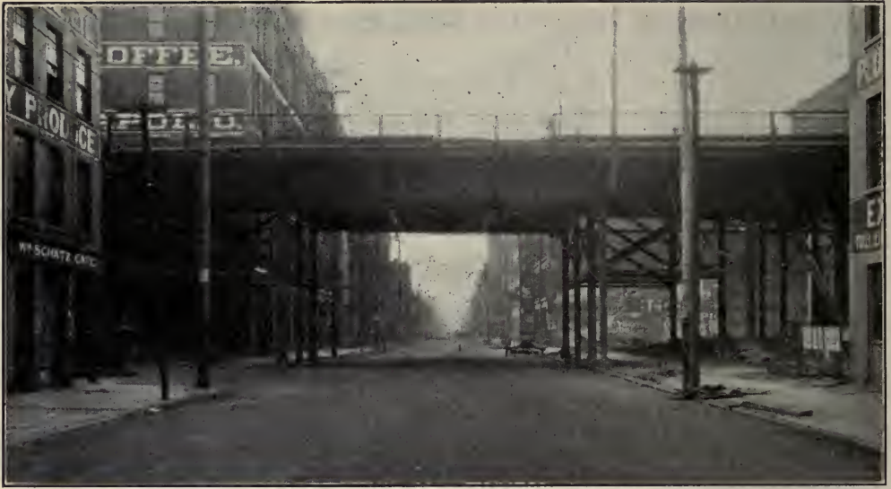
THE FINISHED PAVEMENT ON SECOND STREET, CINCINNATI, OHIO
